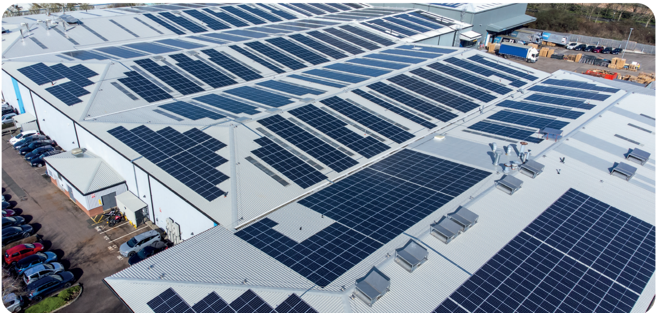
Image: Solar photovoltaic (PV) units on the roof of Thorlux's manufacturing facility
